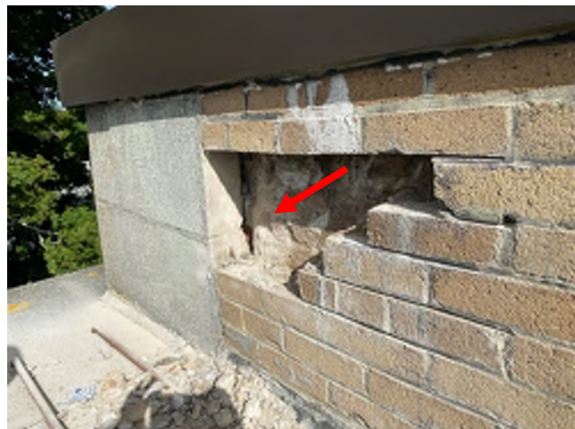
Image 254: View of brick masonry test cut no. 2.
