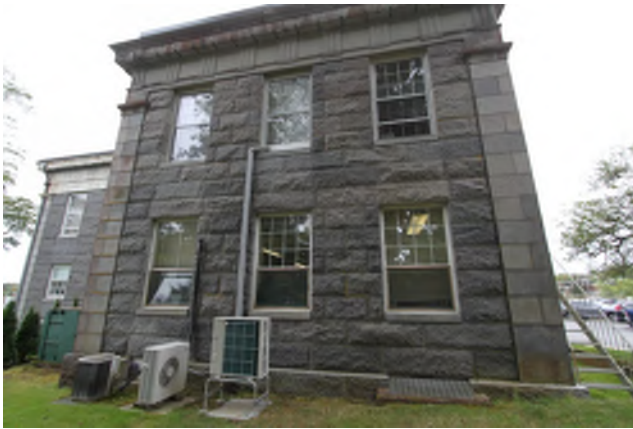
Image 162: West elevation of the 1925/26 wing.
