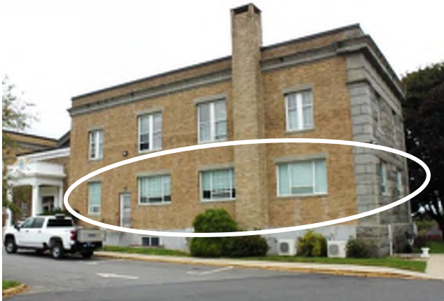
Image 25: Overall view of the South Elevation of one of the 1925 Addition wings. Steel windows are typically installed on the first floor of these wings (circle).
