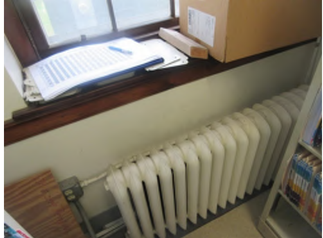
Image 78: View of the window sill within the stacks room.
