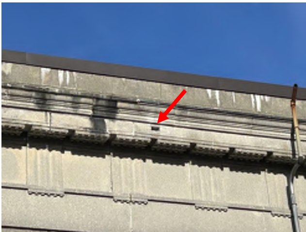
Image 255: View of precast concrete test cut no. 1.
