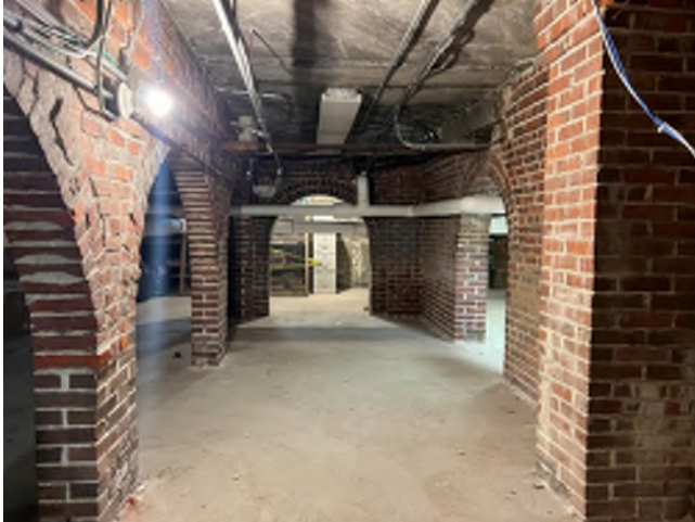
Image 225: Partial overall view of the masonry piers in the basement of the 1831-1832 building.
