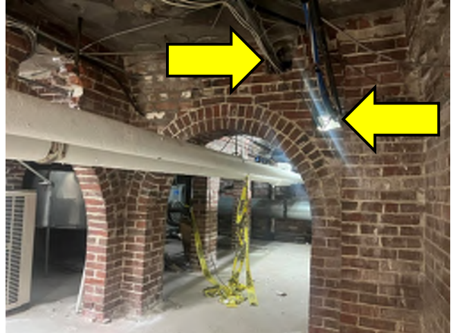
Image 230: View of the two (2) voids above the masonry arch where electrical conduits were installed.
