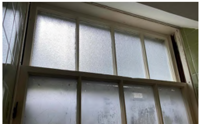
Image 16: Basement windows within bathrooms either utilize obscured, textured glass or a translucent film to reduce visibility.
