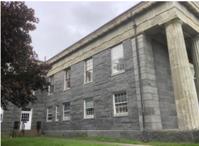
Image 139: Overall East Elevation of the 1832/33 Building.
