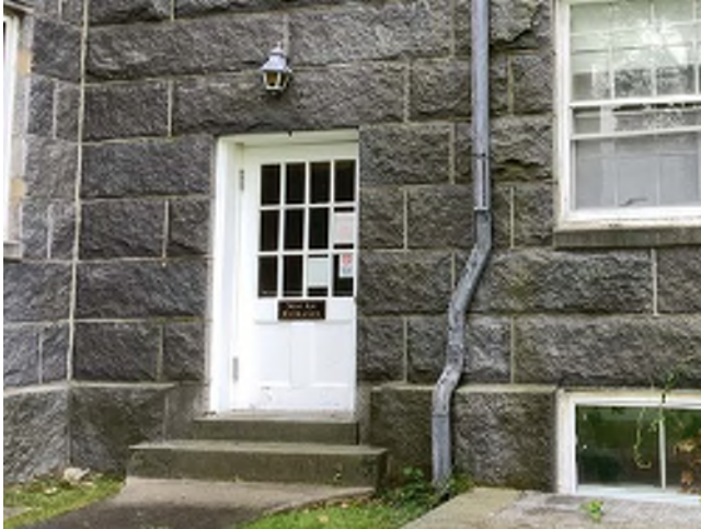
Image 113: Exterior view of Door 4.
