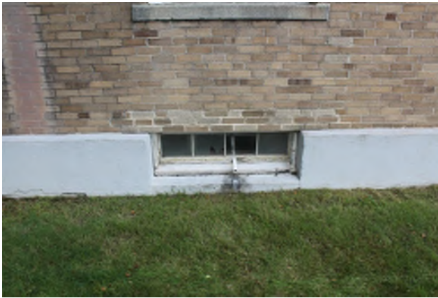
Image 39: Exterior view of one (1) of the wood basement windows.
