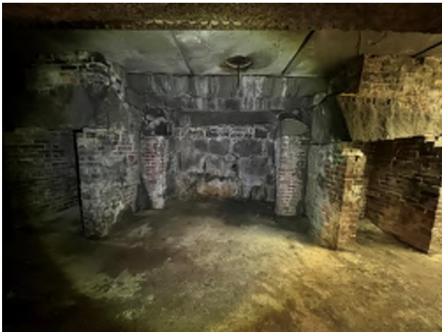
Image 235: Overall view of the north wall below the exterior granite steps.
