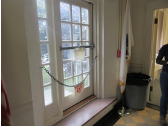
Image 99: Interior view of Door 1.
