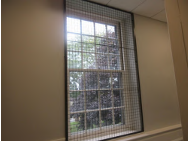
Image 81: View of a typical window within the lock-up area. Interior security screens are installed at the windows within this space.
