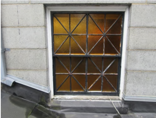
Image 269: Exterior view of a typical double-hung window at the building.
