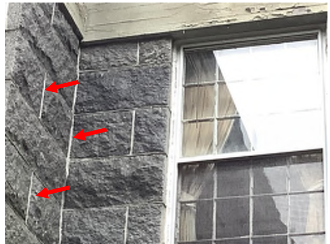
Image 152: View of sealant application over rock-faced granite mortar joints.
