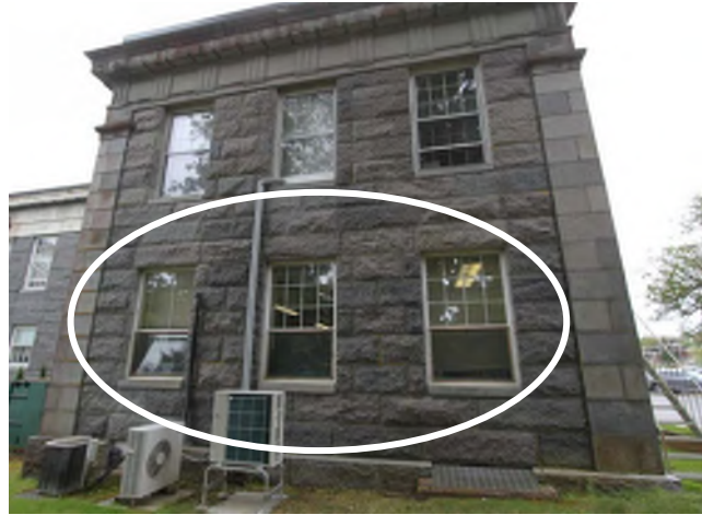
Image 26: Overall view of the West Elevation of one of the 1925 Addition wings. Steel windows are typically installed on the first floor of these wings (circle).
