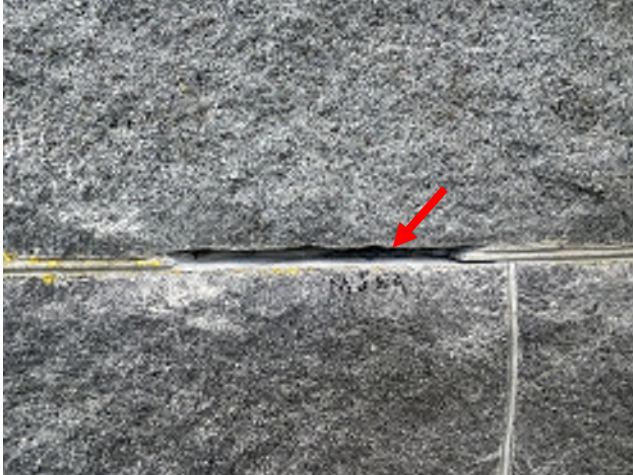
Image 247: View of granite mortar joint test cut no. 4.
