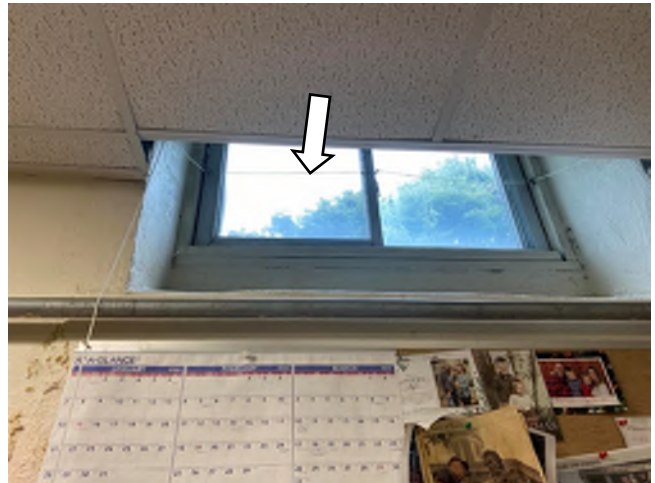
Image 36: Interior view of a typical basement sliding window. The arrow indicates a rope attached to the sliding sashes that appears to be means of operating the windows that are too high to operate manually.
