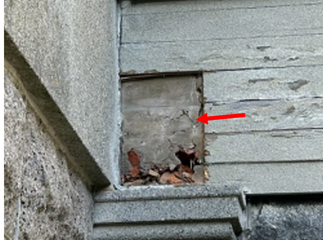
Image 262: Closer view of the previous image shows terra cotta behind painted tongue and groove wood fascia boards.
