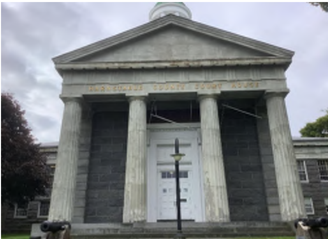
Image 137: Overall North Elevation of the 1832/33 Building.
