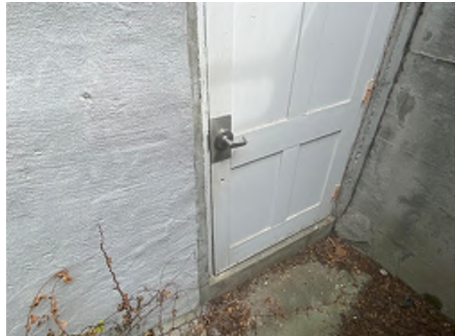
Image 128: Exterior view of Door 7 and threshold. The door threshold is raised above the interior floor and exterior landing levels.
