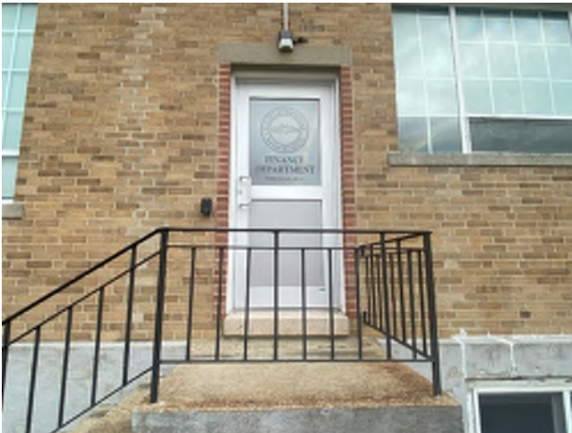
Image 131: Exterior view of Door 9 and associated portico.
