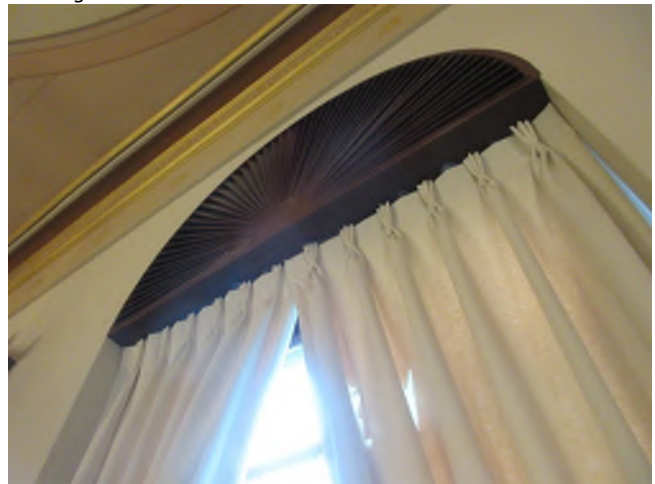
Image 56: View of the typical fan-like arched wood transom and drapes at each window within this space.
