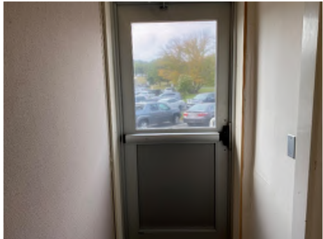
Image 132: Interior view of Door 9.
