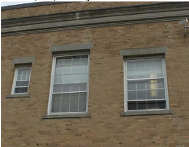
Image 23: Detail view of typical double-hung wood windows at the 1925 Addition.
