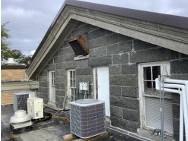
Image 17: View of windows and door located above roof line on the South elevation.
