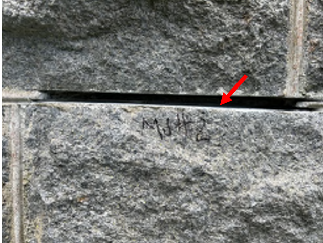
Image 243: View of granite mortar joint test cut no. 2.
