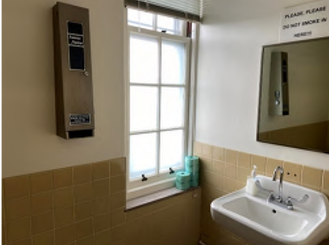
Image 85: One (1) example of a window opening divided by an interior partition wall.
