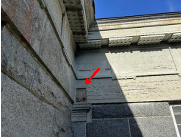
Image 261: View of wood test cut no. 1, which was performed directly above a granite pilaster.
