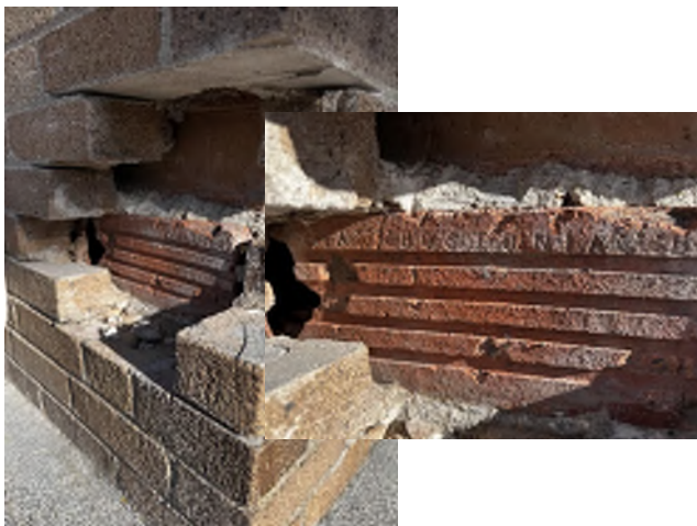
Image 253: View of brick masonry test cut no. 1 shows terra cotta backup.
