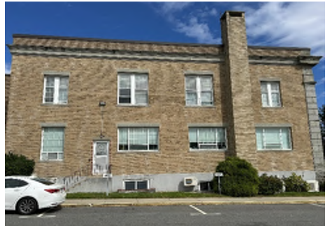
Image 171: View of the east wing of the south elevation on the 1925/26 addition.
