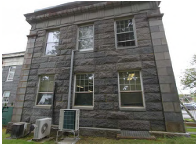
Image 22: Overall view of the West Elevation of one of the 1925 Addition wings. Wood windows are typically installed on the second floor of these wings.
