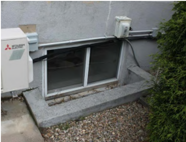
Image 35: Exterior view of a typical basement sliding window
