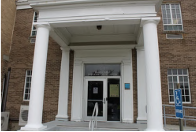
Image 129: Exterior view of Door 8 and associated portico.
