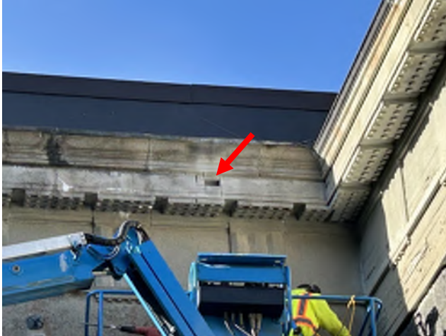
Image 257: View of precast concrete test cut no. 2.
