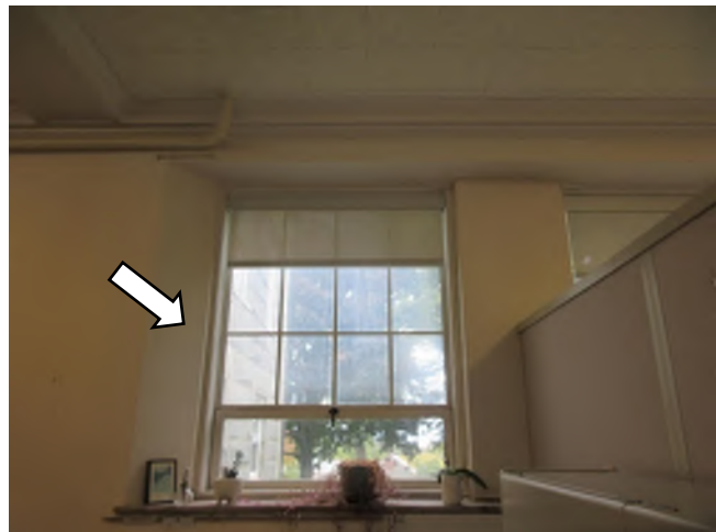
Image 64: The arrow indicates an example of a window with an angled jamb.
