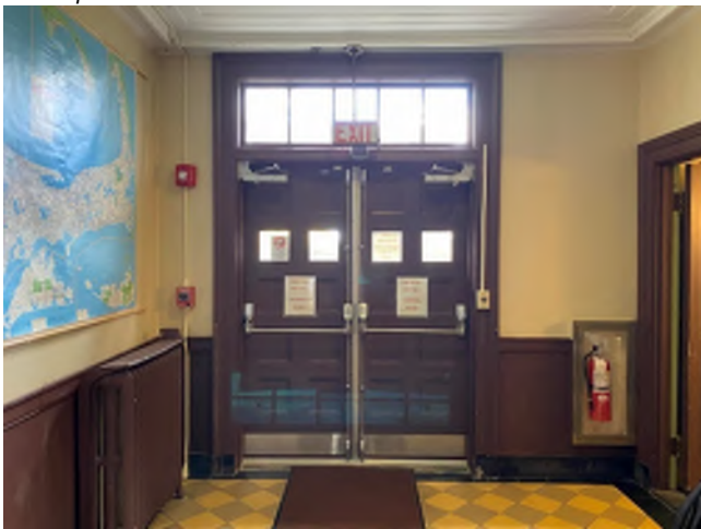
Image 109: Interior view of the Door 2 threshold.
