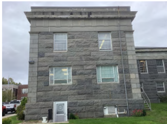
Image 157: East elevation of the 1925/26 addition.
