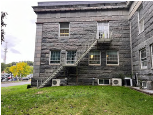
Image 239: Overall view of the fire escape located at the east elevation of the 1893/1906 addition.
