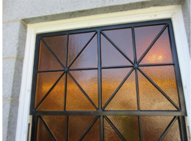
Image 274: Eventually the windows received finish paint and were reinstalled.
