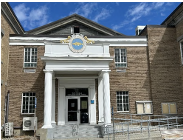
Image 198: Overall south elevation of the 1971 addition shows brick masonry and wood elements around the main entrance.
