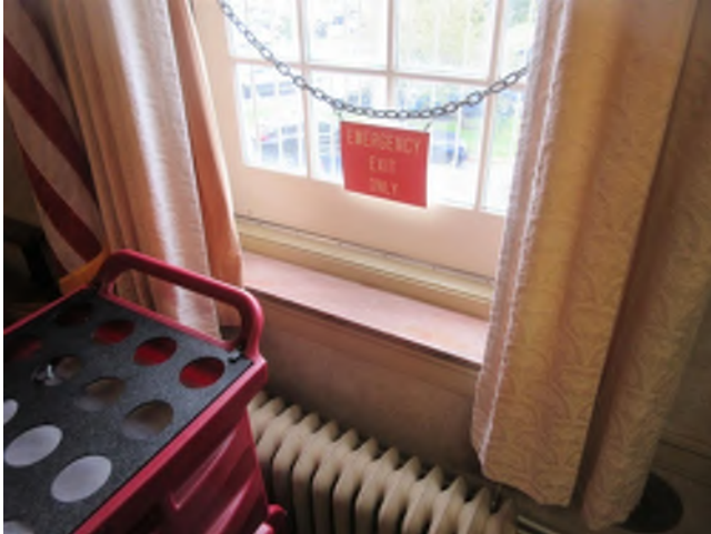
Image 121: The door is raised above the interior floor level.
