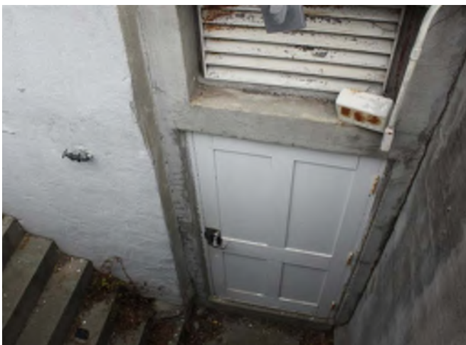
Image 123: Exterior view of Door 7 with louver above.
