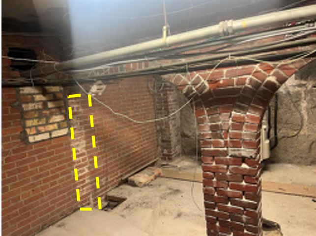
Image 233: Overall view of masonry arch where the masonry pier was removed. Refer to Image 10 for a closer view of the masonry pier that was removed. Note: The dashed box indicates the approximate location of masonry pier.
