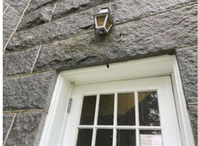
Image 114: Exterior view of Door 2 and transom.
