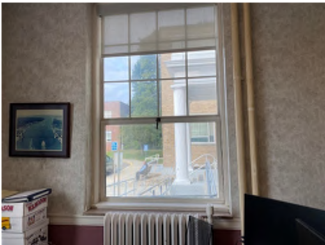
Image 63: View of a typical window opening within this space.
