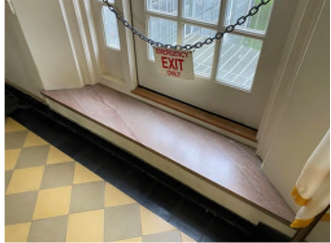
Image 100: A marble stool is installed on the interior side of the door, similar to the windows.
