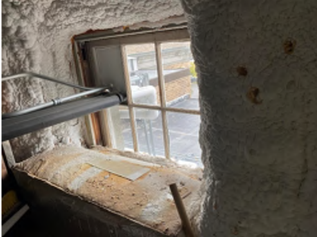
Image 97: Interior view of one (1) of the attic windows, with spray foam installed into the window opening returns.
