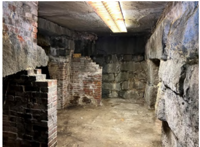
Image 236: Overall view of the east wall below the exterior granite steps.
