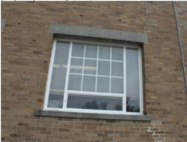
Image 27: Typical large steel window opening, with center hopper unit and fixed lites above and on either side of the hopper unit. Note that the muntins are only installed at the fixed lite above the hopper unit at this location. The insect screen is also missing from this window location.
