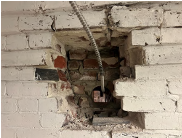
Image 231: View of two (2) wythes of brick removed and a hole cored in the third wythe to install an electrical conduit in the basement wall.
