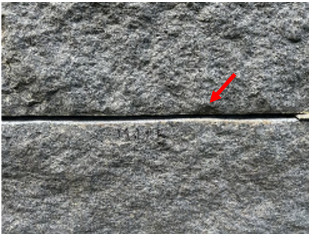
Image 249: View of granite mortar joint test cut no. 5.
