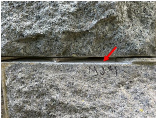
Image 241: View of granite mortar joint test cut no. 1.
