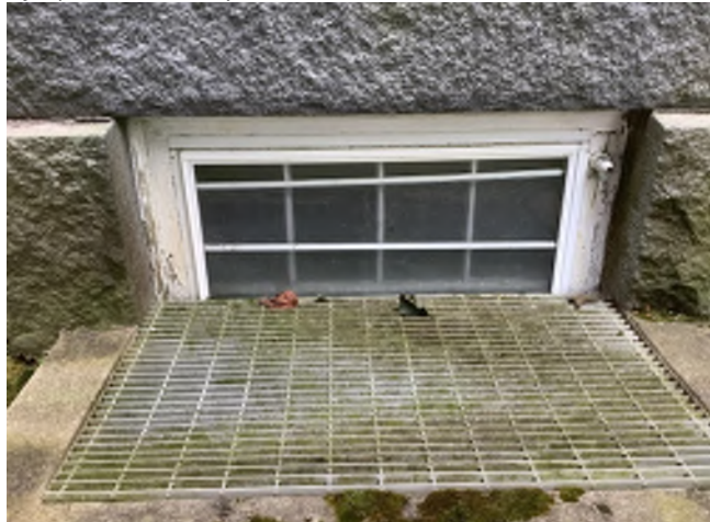
Image 4: Typical Basement window within the 1893 and 1903 wing additions.
