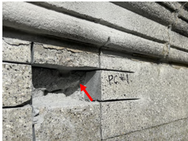
Image 256: Closer view of the previous image shows precast concrete that appeared intact.
