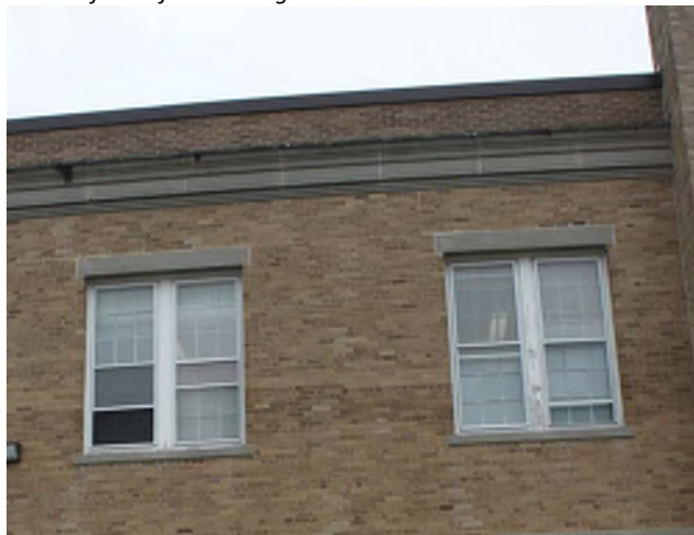
Image 24: A number of the openings at the 1925 Addition feature a wood-framed center mullion.
