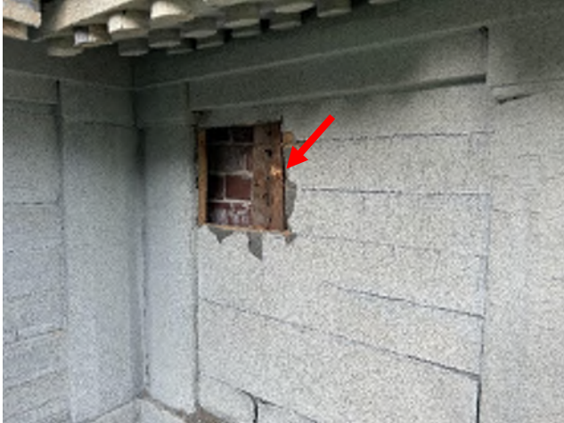
Image 265: View of wood test cut no. 3 shows painted wood fascia on wood furring against brick masonry.
