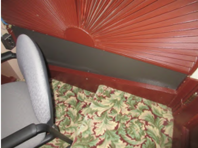
Image 53: On the opposite side of the mezzanine, the window has been provided with a dark colored blank-off panel.
