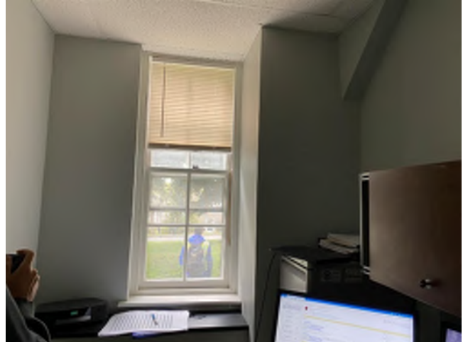
Image 70: An additional example of a window opening within the 1832 first floor offices.
