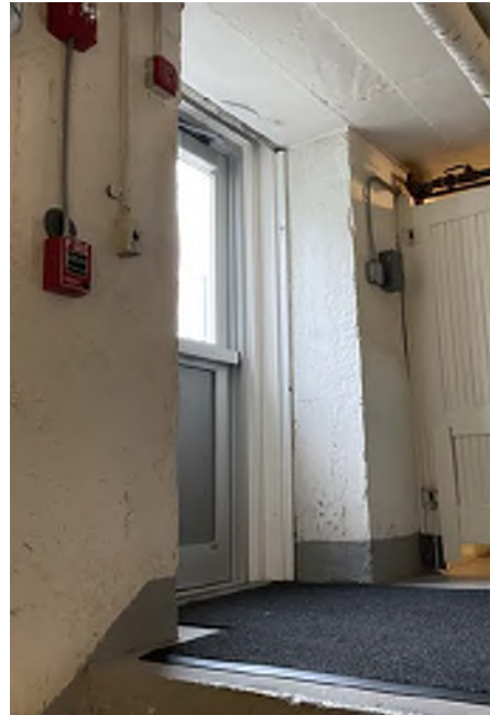
Image 118: Exterior view of Door 5.
