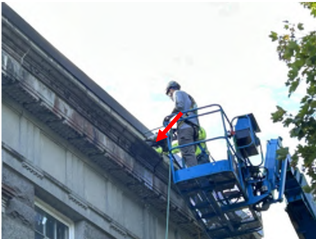
Image 259: View of precast concrete test cut no. 3
