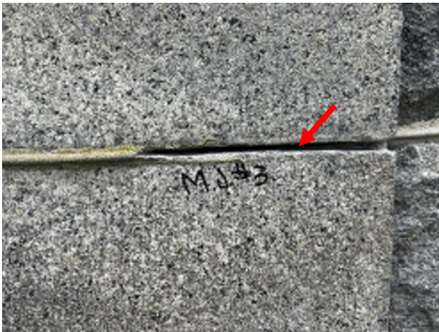
Image 245: View of granite mortar joint test cut no. 3.
