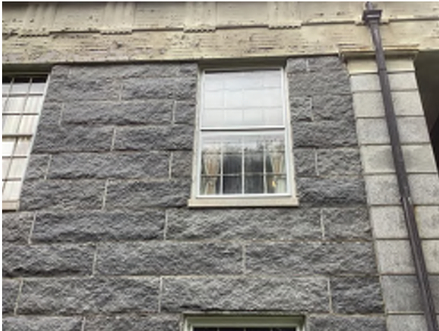
Image 3: Typical Second Floor window at the Original building viewed from the exterior.
