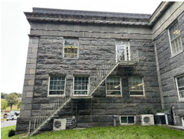
Image 156: North elevation on the east wing of the 1925/26 addition.
