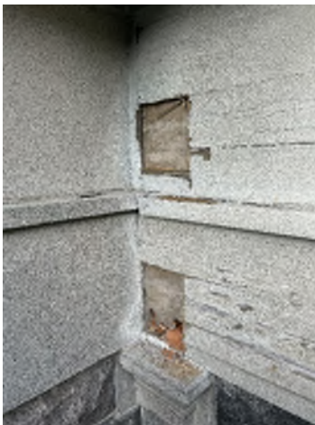
Image 263: View of wood test cut no. 2 depicted by the arrow.
