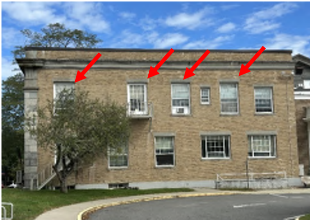
Image 170: View of the west wing of the south elevation on the 1925/26 addition. The arrows identify locations of dissimilar brick masonry units.
