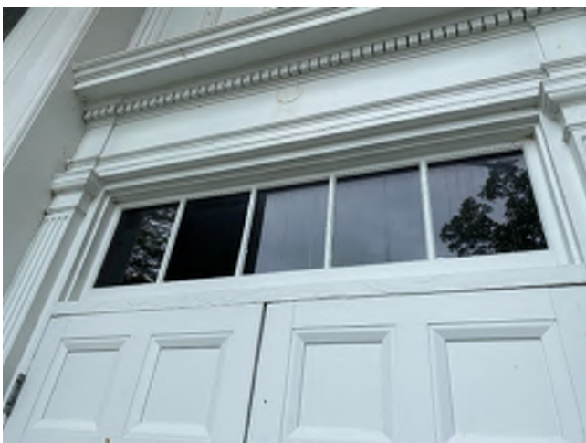
Image 111: Detail view of the door transom.
