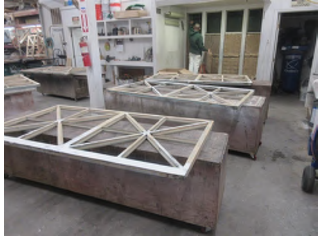
Image 270: Window sashes were removed and transported to a window workshop. The windows were de-glazed and stripped of paint.
