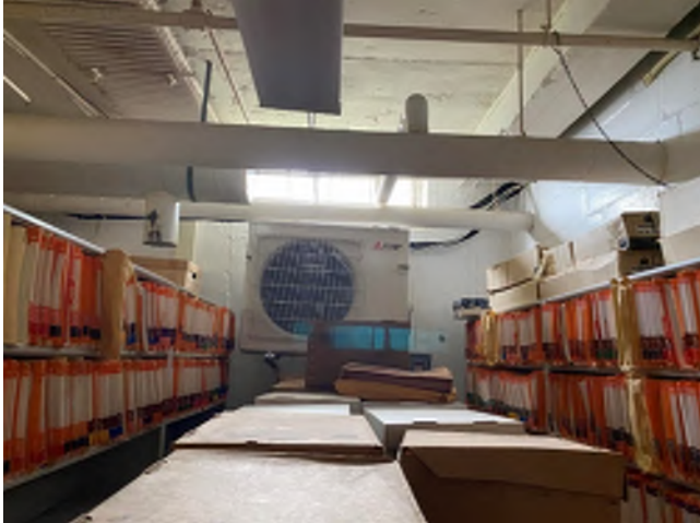
Image 93: View of the storage area in the basement. A split system and multiple shelving units were observed to be installed below one (1) window in this space.
