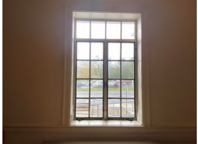
Image 46: Interior view of a typical 1971 Addition steel window.
