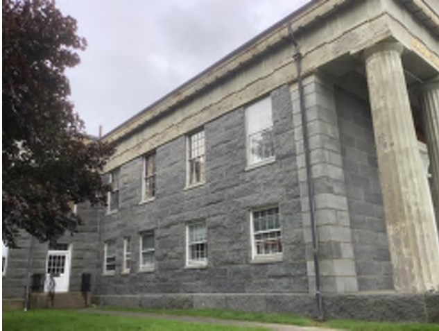
Image 1: Overall view of typical window openings at the Original building.
