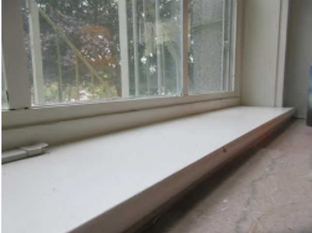
Image 65: View of the typical wood stool installed over the marble stool to the right of the image.
