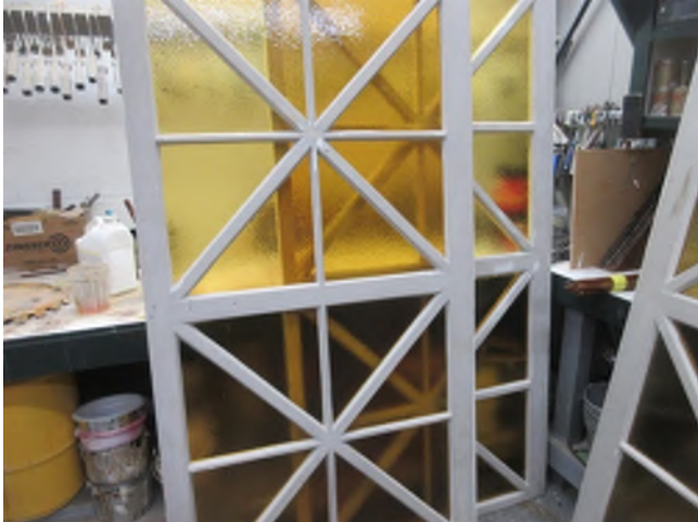
Image 273: Once repaired, the windows were primed and re-glazed.
