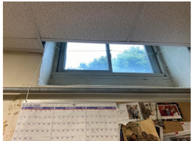
Image 96: Newer aluminum sliding windows within the facilities office are installed above the suspended ceiling level.
