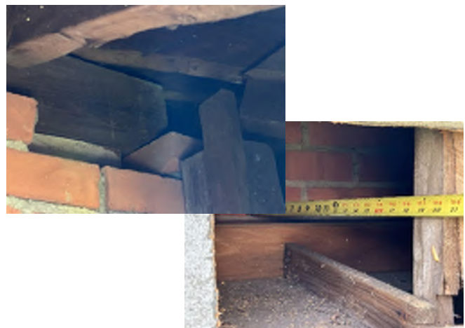
Image 268: A brick masonry wall that extends up to the underside of the roof observed in wood test cut no. 4.
