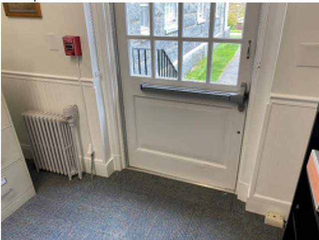
Image 105: Interior view of the Door 2 threshold.
