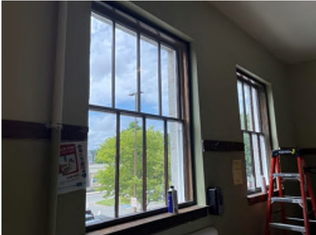
Image 275: Additionally, the client opted to install fixed aluminum storm windows at all openings.
