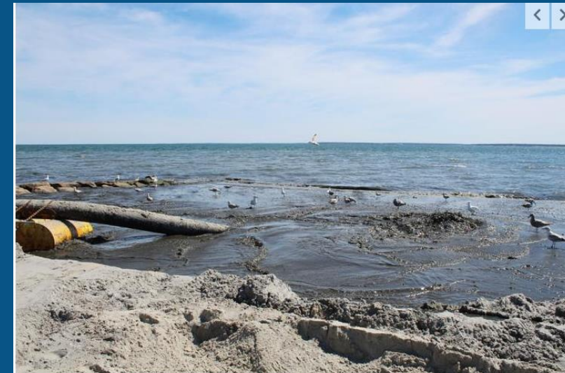
Freshly dredged material poured through the dredge pipe and onto InnSeason Beach. GILDA GEIST/ENTERPRISE
