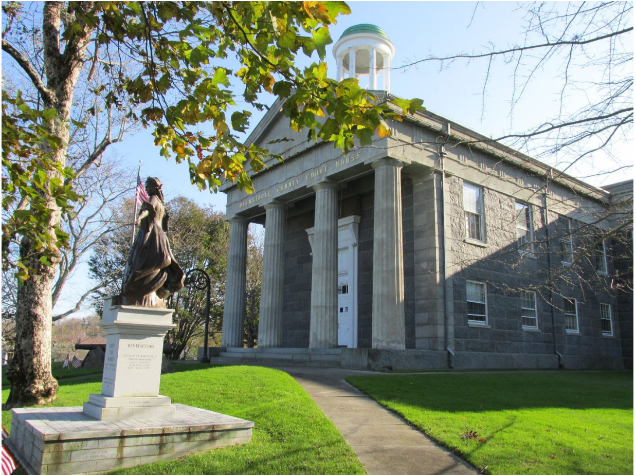
Barnstable County Superior Court House
