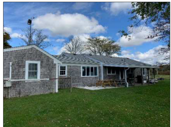
New roof to receive solar panels
