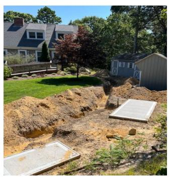
Presenting the completed emergency generator and propane tank pads, complete with the trench for the gas line leading to the main house.
