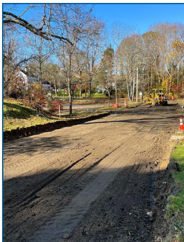
Grading site for new pavement
