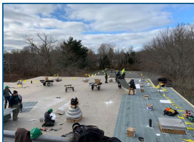
Workers install new insulation and EPDM membrane at Orleans Second District Court
