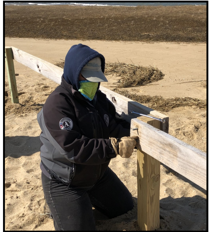
Celia repairs a kayak rack in Wellfleet during the COVID-19 pandemic.
