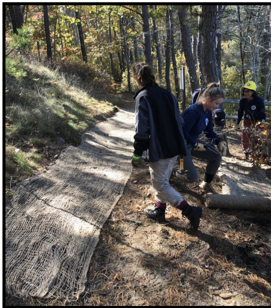
Bee, Katie, and Lourdes install jute to prevent shoreline erosion at Dyer Pond.
