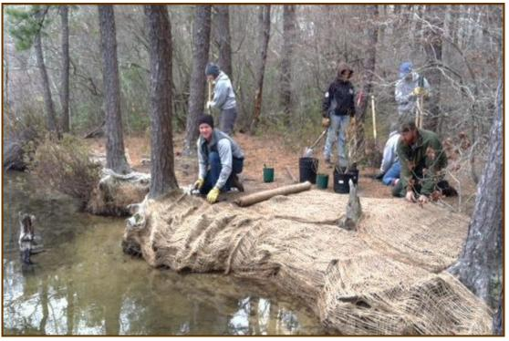
Members install jute netting in order to hold soil in place.
