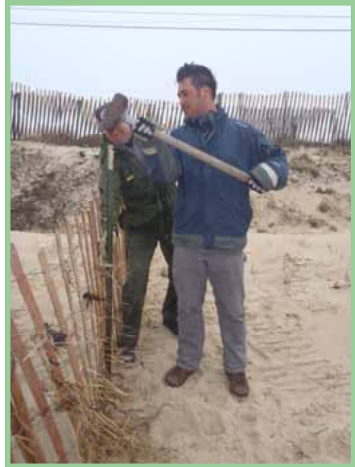
Member Mike Evans works with Army Corps Ranger John Pribilla to install dune fencing.
