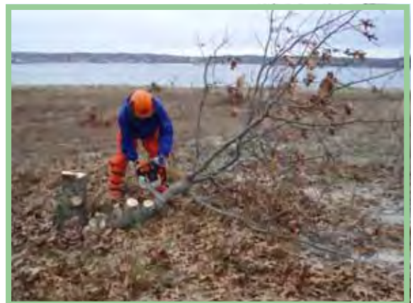
Colum Lang uses a chainsaw to remove woody vegetation from Mashnee Dike in Bourne.
