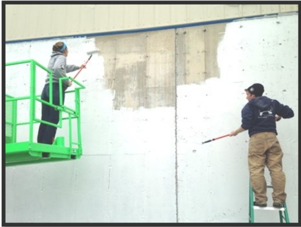
March 11, 2014: The first coat of primer is applied.
