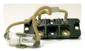
Mercury is also in relay switches in refrigerators, freezers and humidifiers, tilt switches for washing machines, and safety valves as well as flame sensors for any gas appliances. Electric switches (left) contain 30 grams of mercury.
