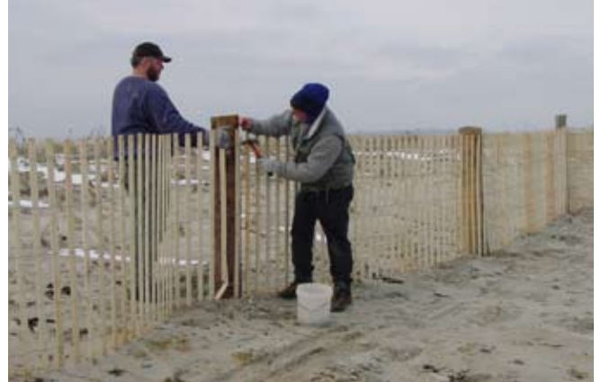
Figure 12. Fence is attached to 6" diameter posts.
