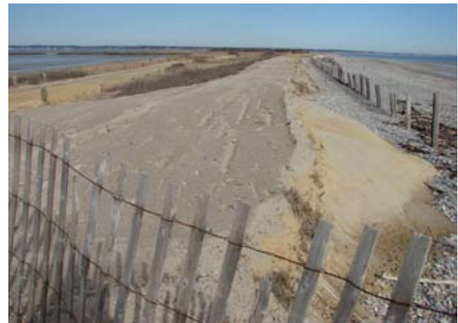
Figure 3. Covering quarry sand with natural dune sand.
