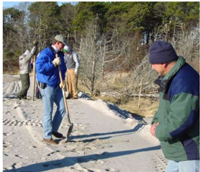
Figure 7. Ted Keon, Director of Coastal Resources for Chatham, Mass., uses a shovel for larger size holes for 6x8 poles while project manager Tim Friary looks on.
