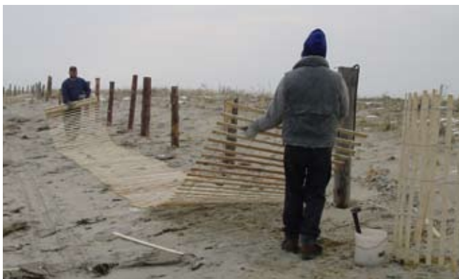
Figure 11. Fence is laid-out.
