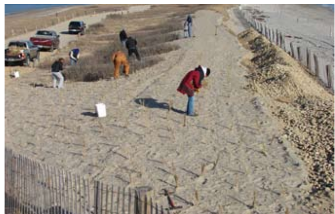
Figure 4. Planting the artificial dune with beachgrass.
