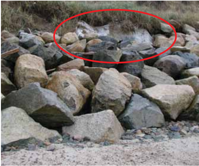
Two examples of geotextiles becoming exposed after erosion, reducing the effectiveness of the shoreline stabilization attempt.
